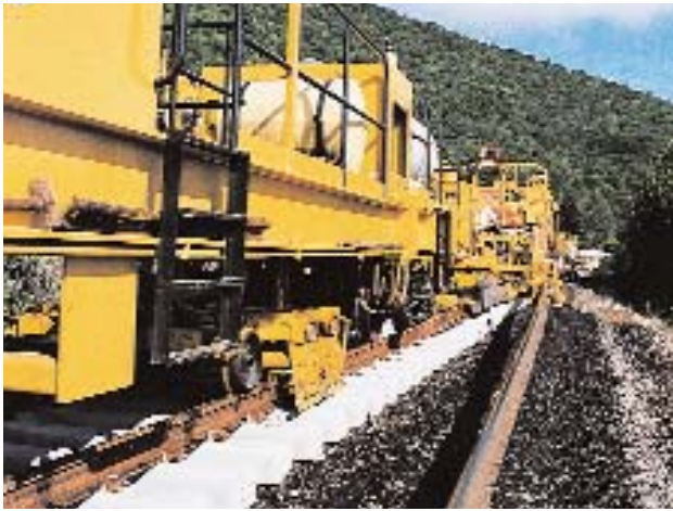
Fairmont Tamper P811 SP-FC installing the PANDROL® FASTCLIP system.
