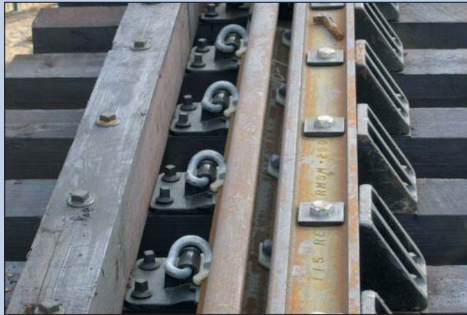
Restraining rail assembly with 115 RE rail.
