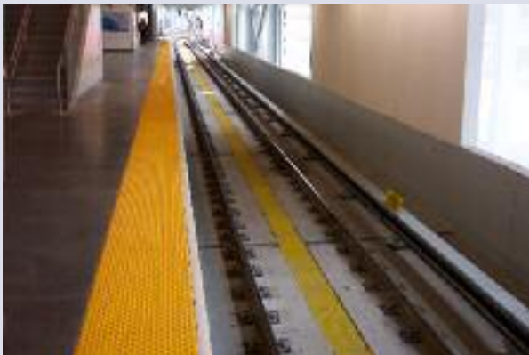
FASTCLIP SRS assembly on slab track
