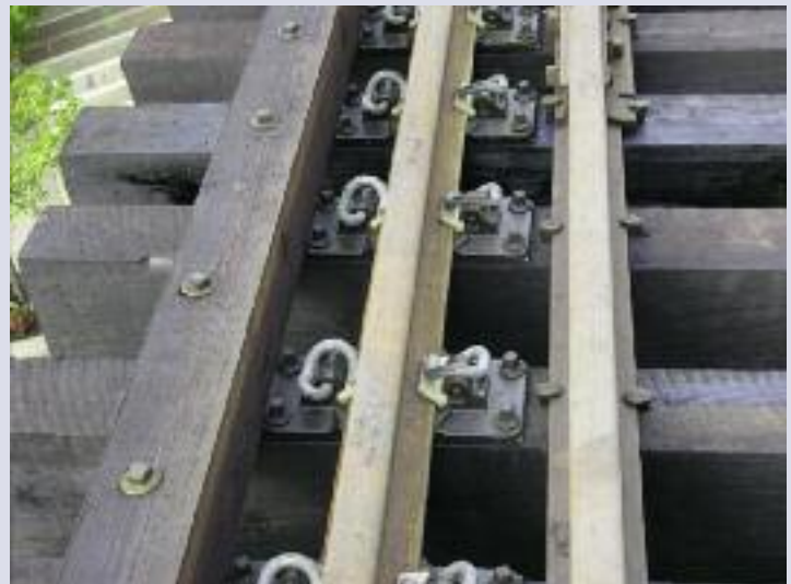
'e' clip SRS assembly (5 1/2" rail base), with 4 holes
