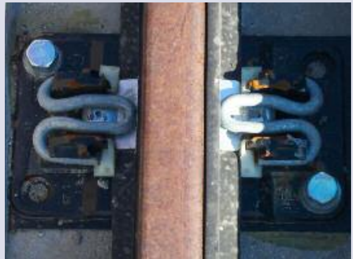
FASTCLIP SRS assembly on slab track
