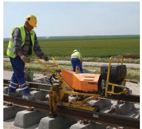
Robel FASTCLIP installation machine
