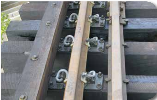
'e' clip SRS assembly (5 1/2" rail base), with 4 holes
