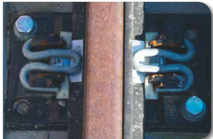
FASTCLIP SRS assembly on slab track
