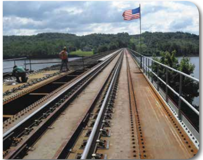
FASTCLIP SRS assembly on a bridge deck
