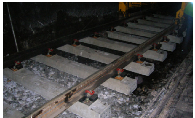
Installation on ballasted track.
