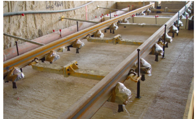
DFF installation Top Down.
