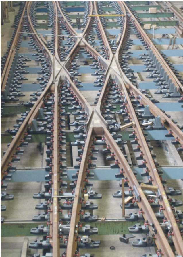
Switches and crossings.
