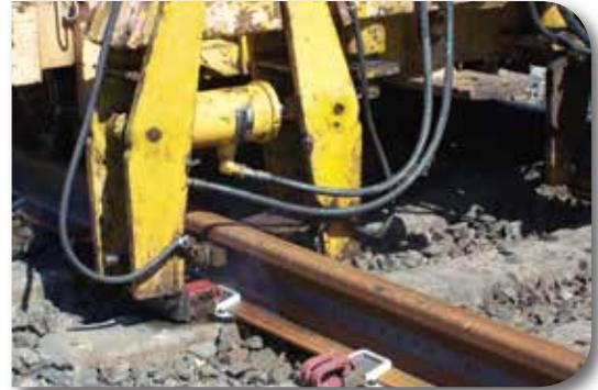
PANDROL Long Reach SAFELOK I clips are available as an option for installations that require a fastening that extends 1/2 inch further on the rail base and generates a slightly higher toe load. This longer reach SAFELOK I fastening has been developed as a safety feature to ensure clip retention and increase holding capabilities on high degree curves where shoulder wear and insulator wear are more prevalent.
