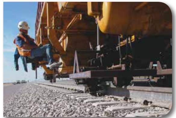
Fast, mechanized application of SAFELOK III
