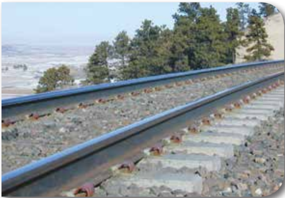
Completed SAFELOK III track
