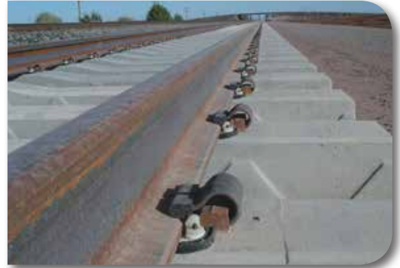
SAFELOK III on recently laid track
